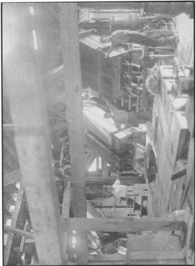
PLATE XVII.—Bromine Stills and Condenser Boxes, Ohio River Salt Corporation, Mason City, W. Va.—This is a wider view of stills shown in Plate XVI.—Photo by courtesy Norman O. Wein.
