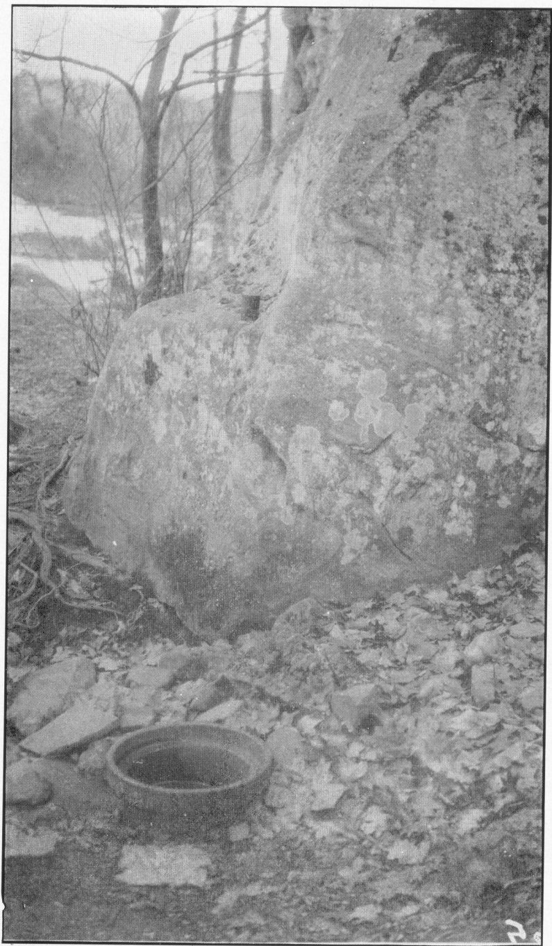
PLATE XX.—The Old Brine Well, Sago, Upshur Co., W. Va.—Drilled by a “sweep” about 1847 and supplied brine for salt for some time. Later was deepened and oil was encountered; finally plugged off below a “flow” of fresh water. In domestic use ever since.—Photo by Hoskins, 1937.
